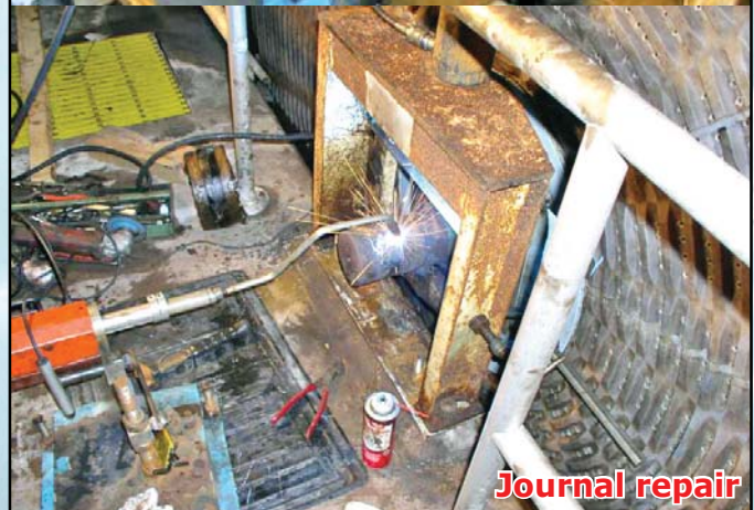
Bore and Shaft Welding
