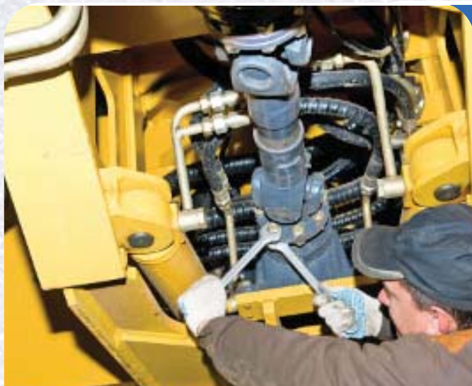
Maintenance & Repair Area
