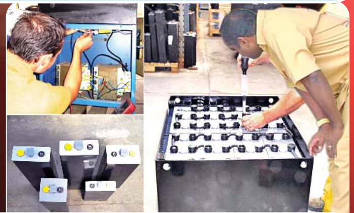
Forklift Battery Cells Replacement
